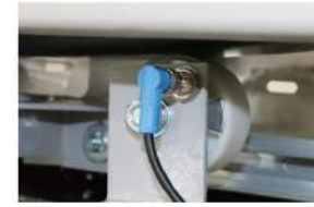
扶手测速 Handrail speed detect
